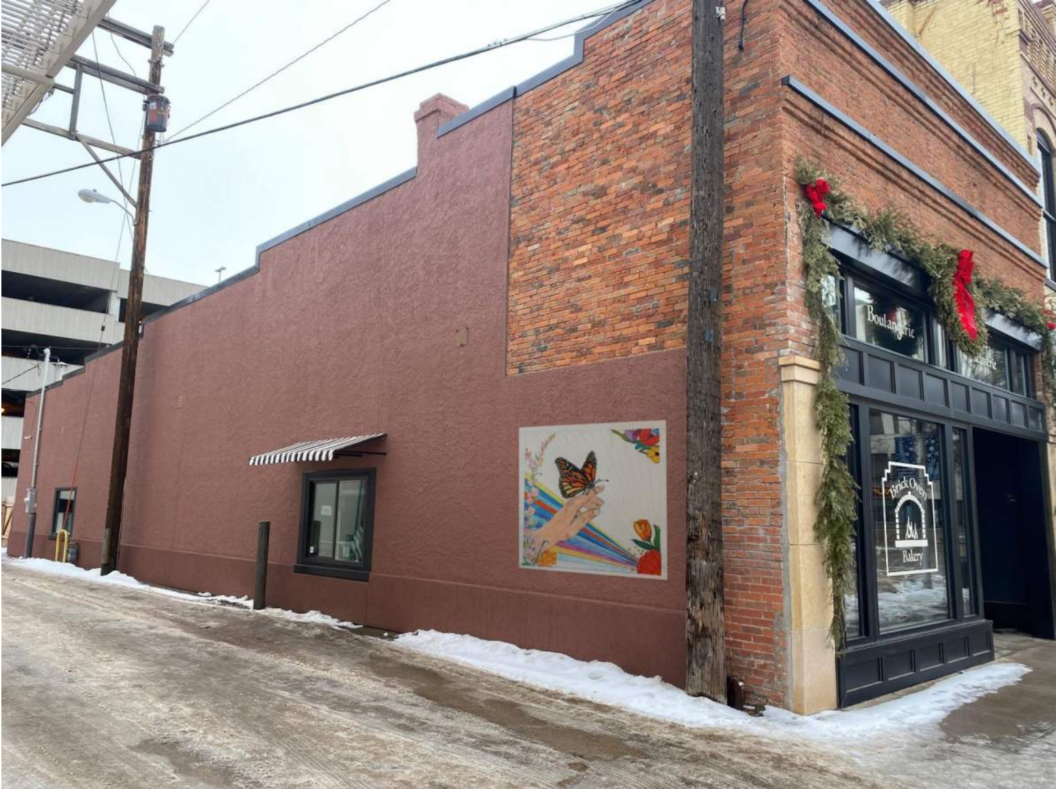
Submitted Design in Approximate Location on South Wall of 112 N 4 th Street
